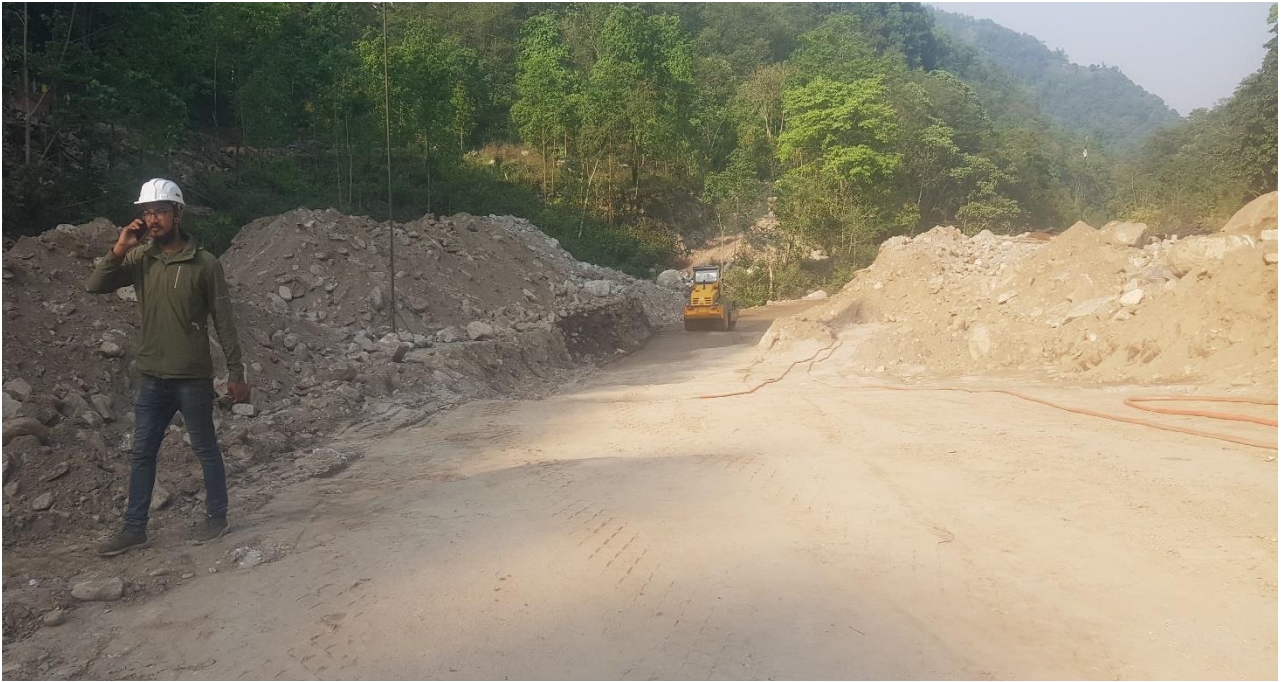
Figure 4: Earthwork in filling and compaction using roller around desander area.
