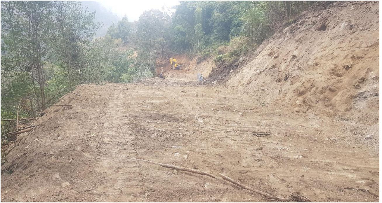
Figure 17: Road widening for Pipeline alignment.
