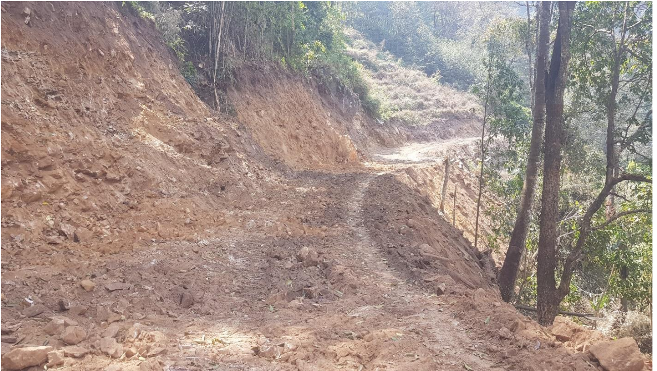
Figure 15: Road Widening for pipeline alignment.
