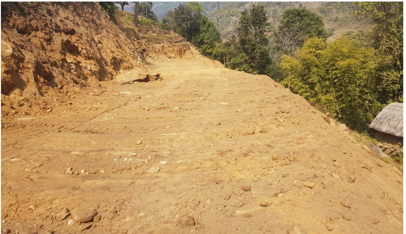
Figure 18: Road Widening for Headrace Pipeline Alignment
