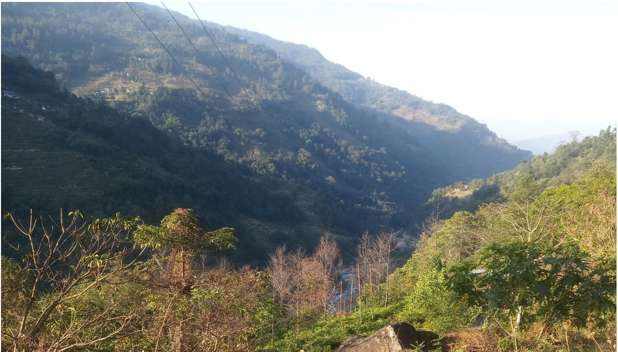
Figure 14: 11 KV Transmission Line for construction power
