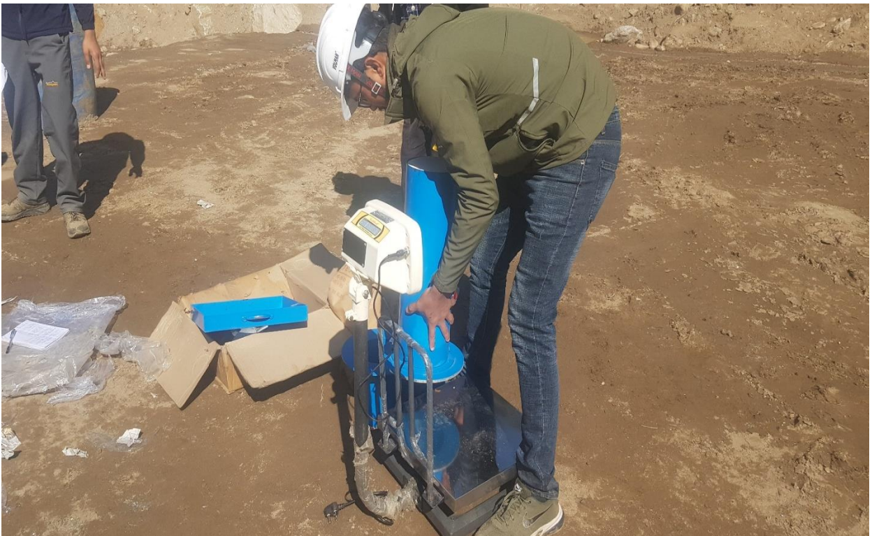
Figure 5: Compaction Testing In desander area.
