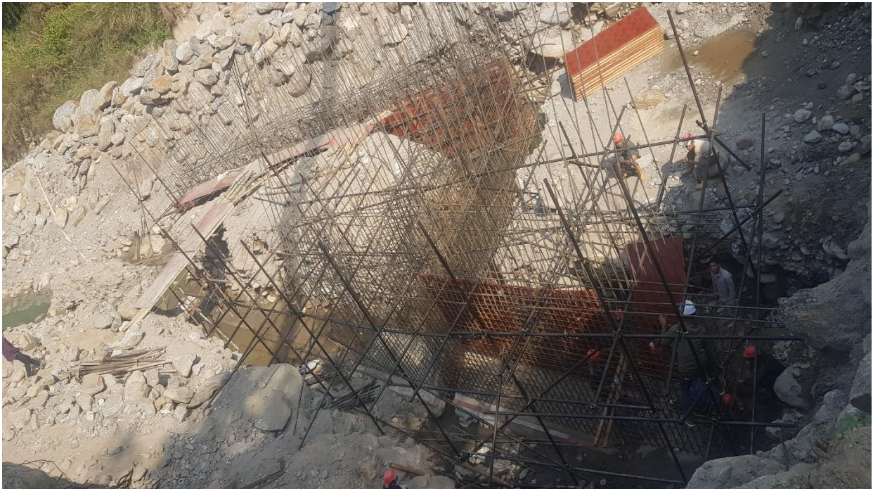
Figure 1: Rebar and formworks installation at divide wall and guide wall
