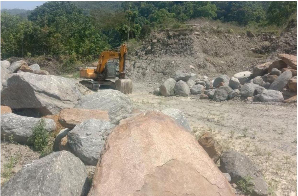
Figure 20: Excavation for Powerhouse Structures.
