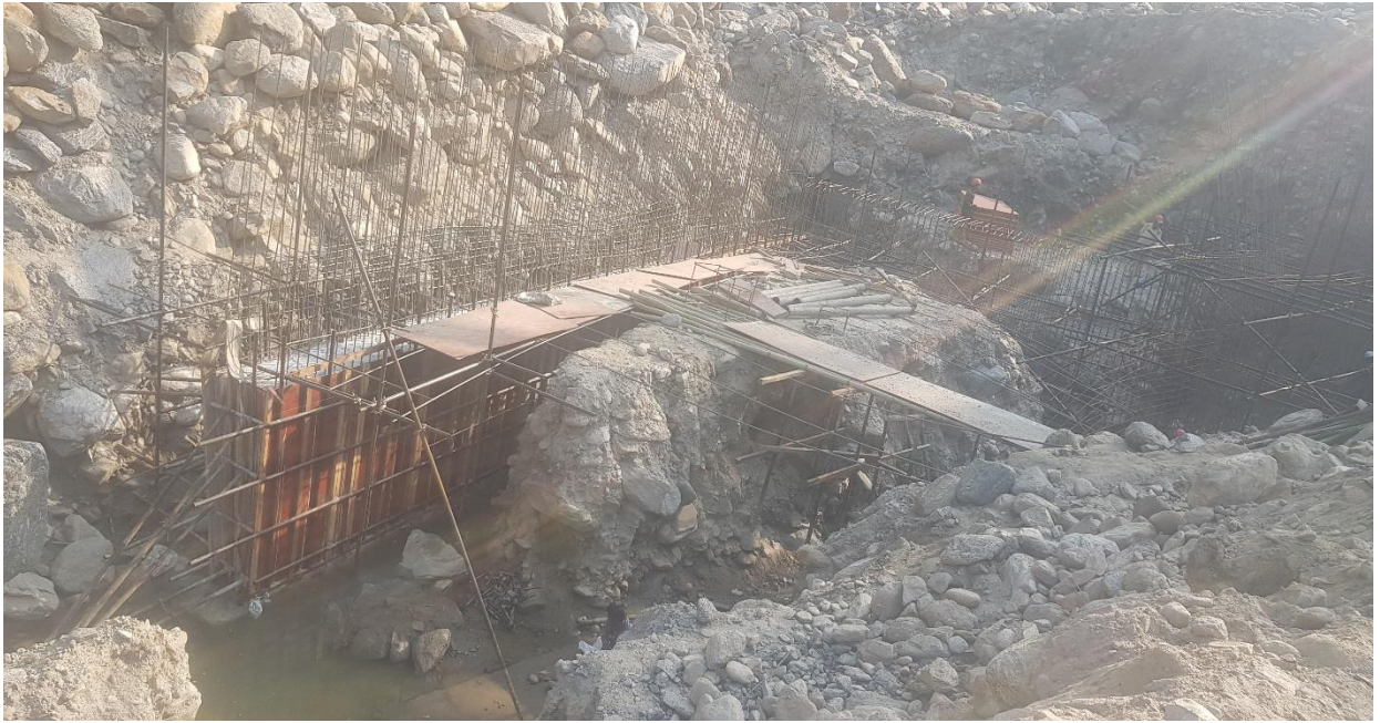
Figure 2: Cutoff Concreting work at headworks.
