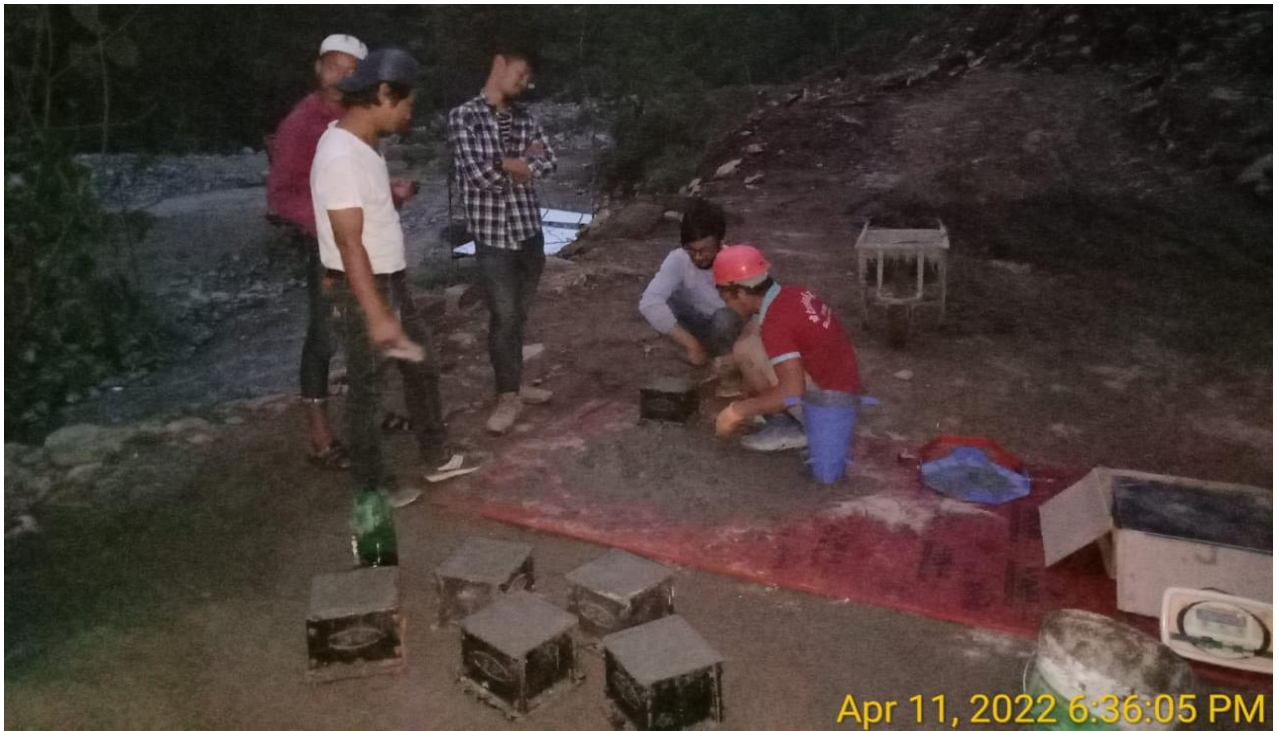
Figure 7: Cube casting for in-site cube casting work.
